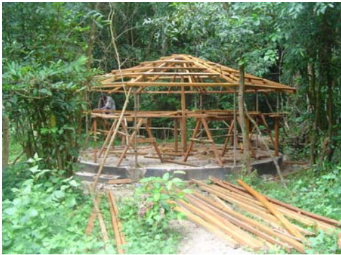
Construction of 5 roofed platforms has been completed to accommodate tents and raised significantly from the ground so as to deter the large number of timber eating termites.
