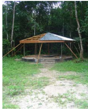
Construction of 5 roofed platforms has been completed to accommodate tents and raised significantly from the ground so as to deter the large number of timber eating termites.
