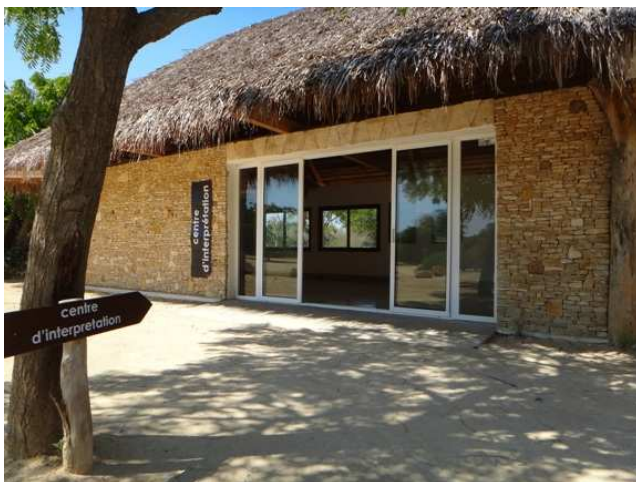
External view of the education centre
