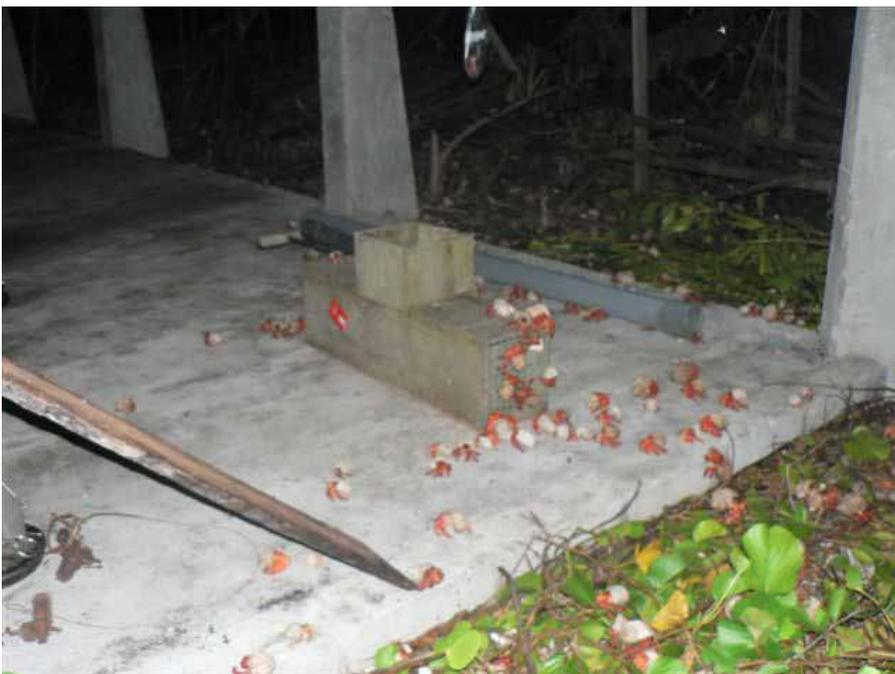
**FIGURE 6.9** – Chimney box and ramp showing crab exclusion.
