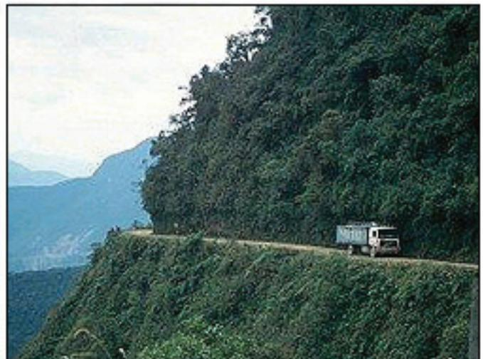
**Old road to the lowlands. The geological instability of the slopes where it was built result in a countless number of landslides. The same fate probably awaits the new road. Photos: Left: SP; Right: MSC**
